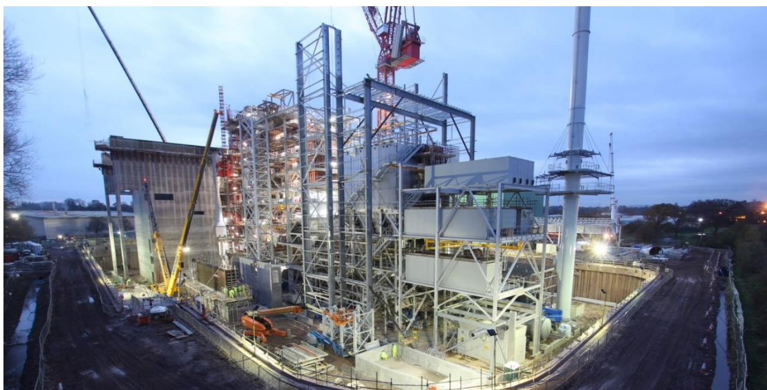
Envirecover Energy from Waste facility under construction.
